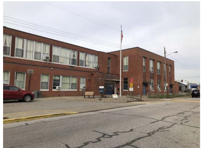
Bridgeview Elementary School
