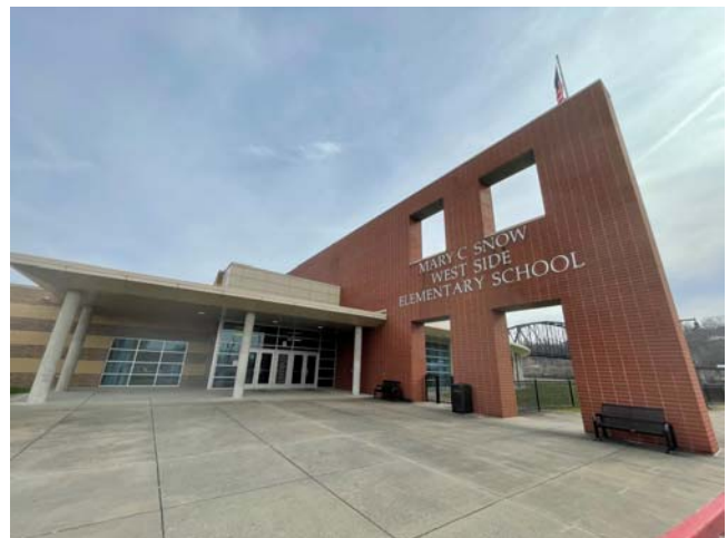
Mary C. Snow West Side Elementary School
